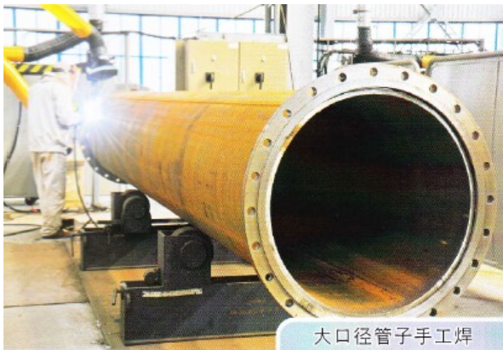
Manual welding of large diameter pipe
